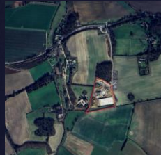
BARSHAM WATER TREATMENT WORKS
